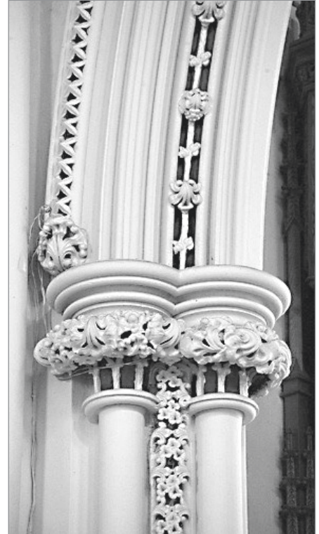
FIG. 32. HAMILTON, CHRIST'S CHURCH, CHANCEL ARCH, DETAIL, NORTH. | MALCOLM THURLBY.
