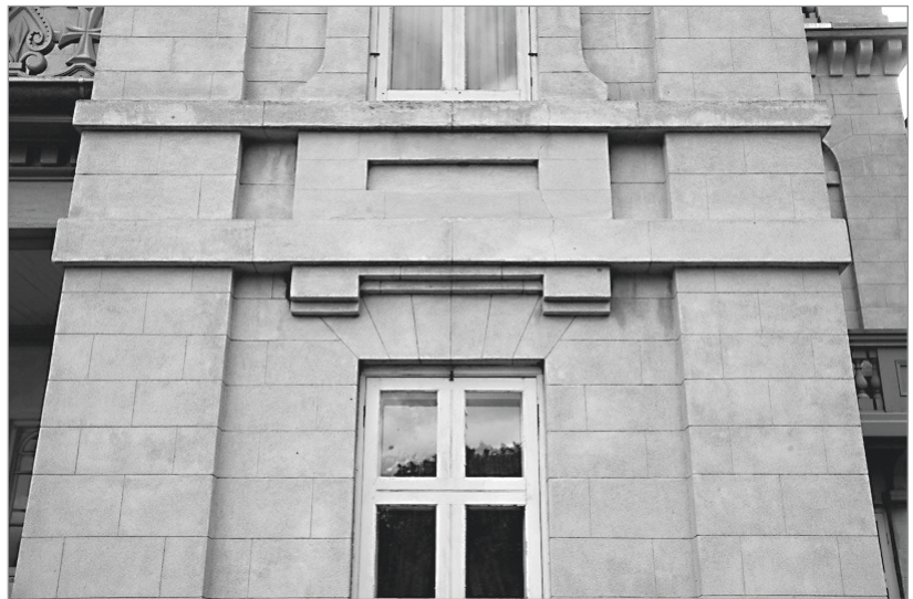
FIG. 10. HAMILTON, DUNDURN CASTLE, IMITATIVE MASONRY DETAIL, ROBERT WETHERELL. | MALCOLM THURLBY.
